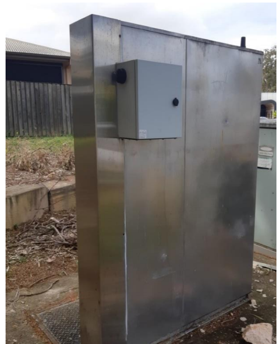
Figure 2 – External lockable installation with stainless steel option. 4G puck antenna on right.
