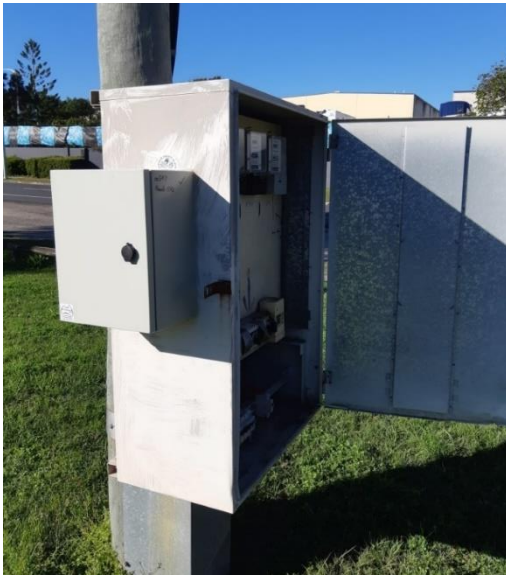
Figure 1 – External Lockable Switchboard Installation
